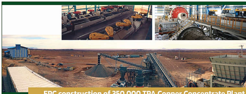
EPC construction of 350.000 TPA Copper Concentrate Plant Abbas Abad Copper Complex, Semnan – Iran
